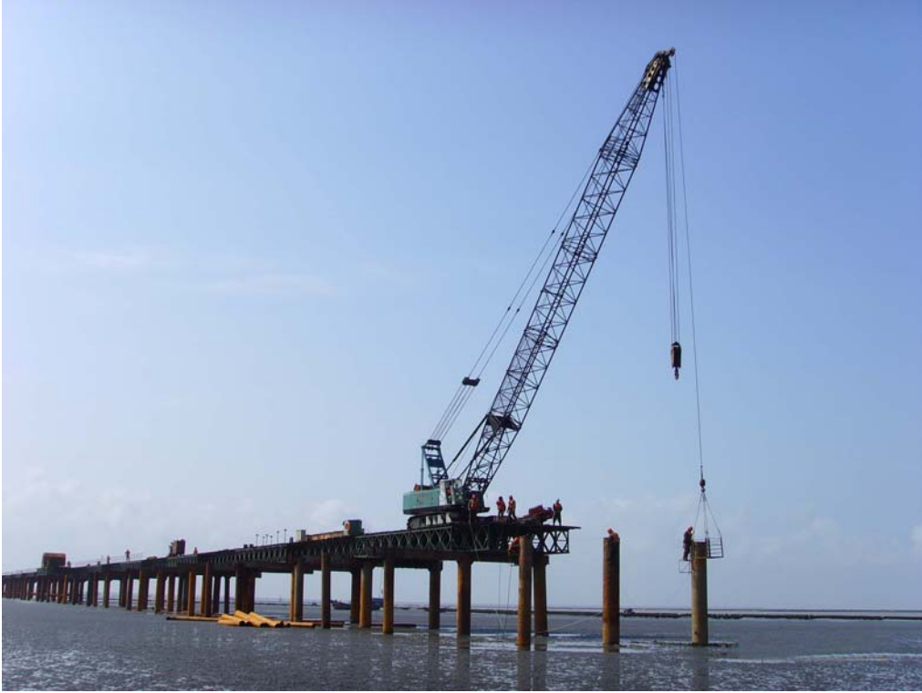
Yellow Sea Crossing Under Construction
